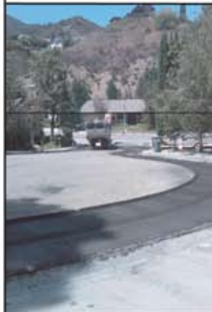
Greenbriar Road Project Mid-Project, July 2009
