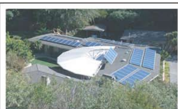
Roof Installation of solar panels.
